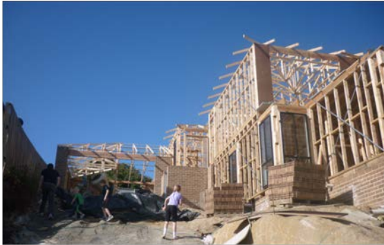
The new house mid-way through construction.
